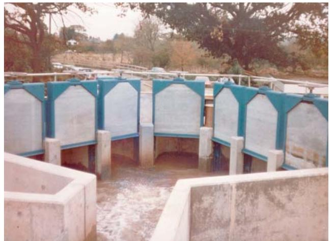
*Coplastix Channel Mounted Sluice Gates*
