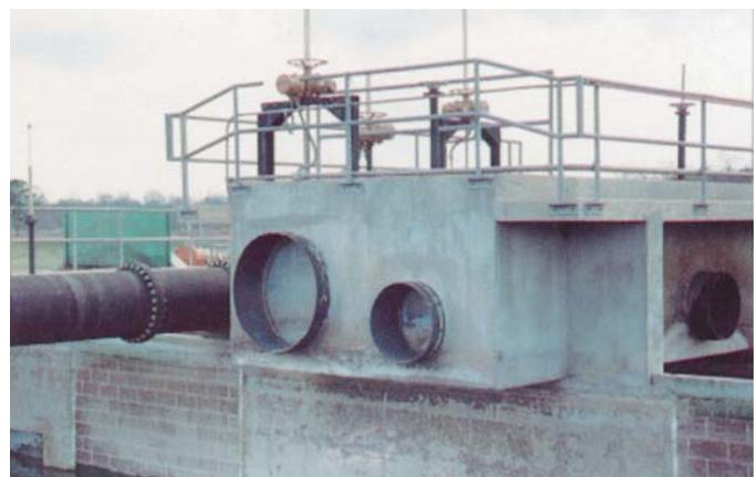
*Coplastix Weir Sluice Gate mounted over circular holes*
