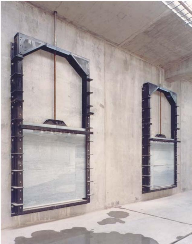
*Coplastix Wall Mounting Sluice Gates*
